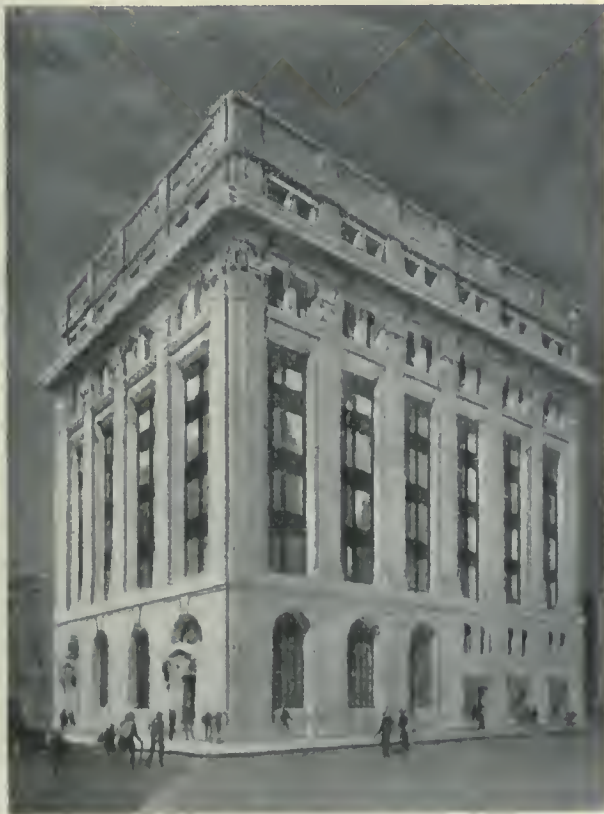
Imperial Oil Building, Church and Court Streets, Toronto.
